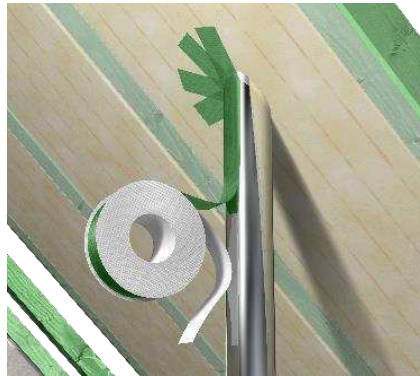
Critical bonding of penetration areas
